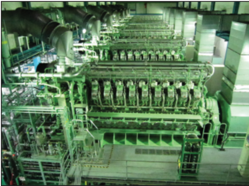
Elpida Memory Inc. recently installed 13 MACH gas engines in their Hiroshima, Japan, factory.
