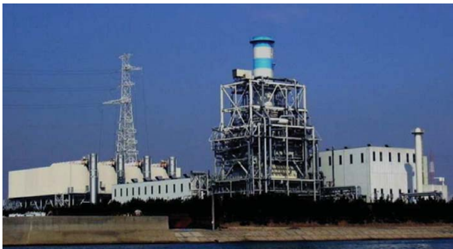
Figure 3: Mitsubishi tests new gas turbine models and components at its inhouse commercial verification facility at Takasago, Hyogo Prefecture
