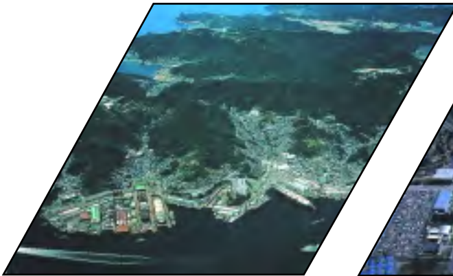
Nagasaki Shipyard and Machinery Works: Boilers, HRSGs, Wind and Steam Turbines
